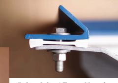
(Left, and above) **Trueseal** is made of PVC material in two different durometer shores to help prevent protrusion.
